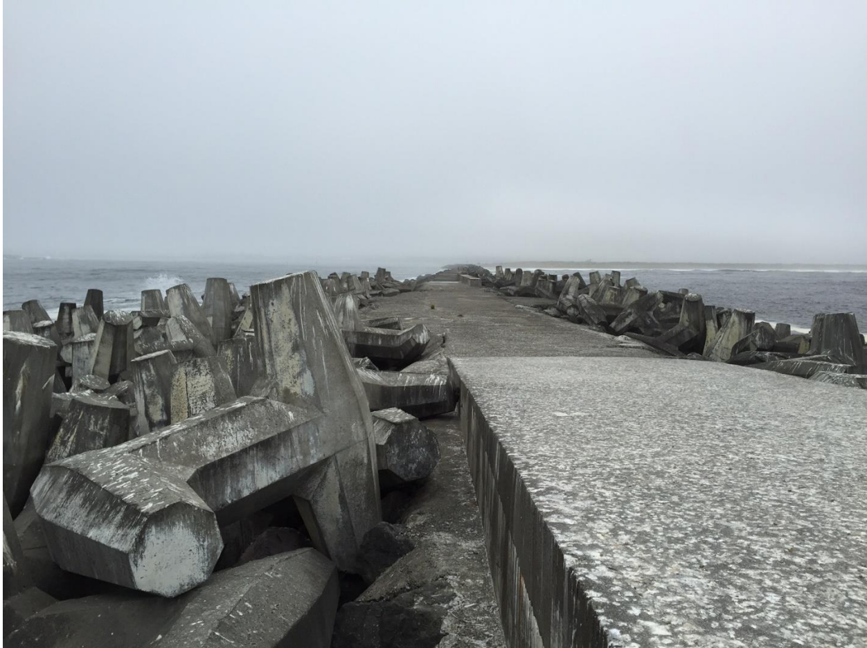
Figure 11: View from the head section of the South Jetty toward the shoreline (August 2016). This area was extensively repaired in the early 1970s. Note the extensive coverage of 42 dolosse and high crest elevation.
